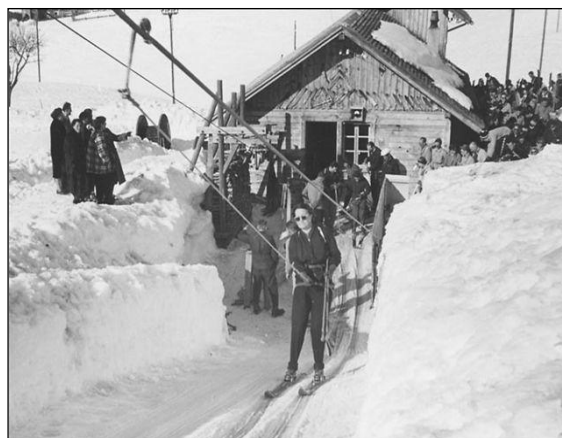
Under the pull, the clamping effect on the circulating steel cable is achieved: off they go!
