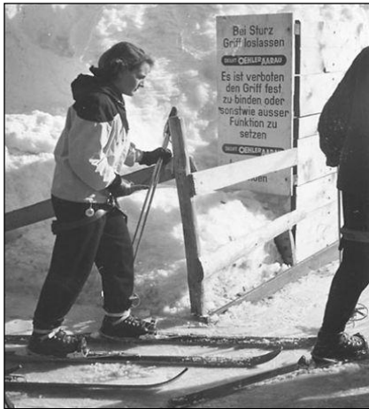
Left: the skier arrives with the belt on, holding the hand grip open, ready to be hooked to the pulling rope. The board warns: “In case of fall, let the hand grip loose. It is forbidden to tie-up the grip or to put it out of function”
