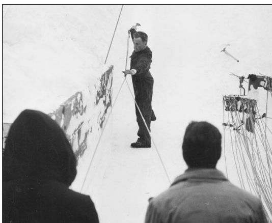
The attendant prepares to hook the rope to the circulating steel cable
