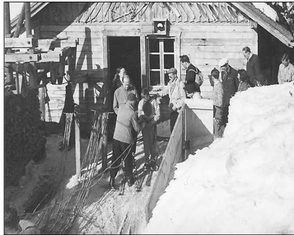
Left: the skier arrives with the belt on, holding the hand grip open, ready to be hooked to the pulling rope. The board warns: “In case of fall, let the hand grip loose. It is forbidden to tie-up the grip or to put it out of function”
