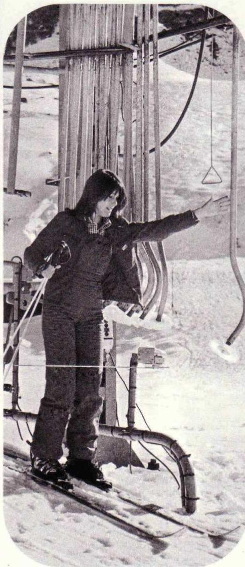
of departure of skiers is regulated by means of either a stop barrier, or green and red signal lamps. Such an automatic departure system permits an economy of staff
